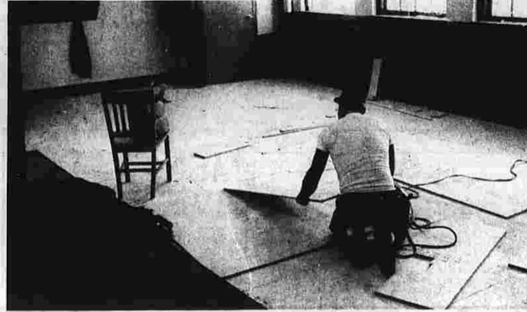
Repairing Storm Damage
